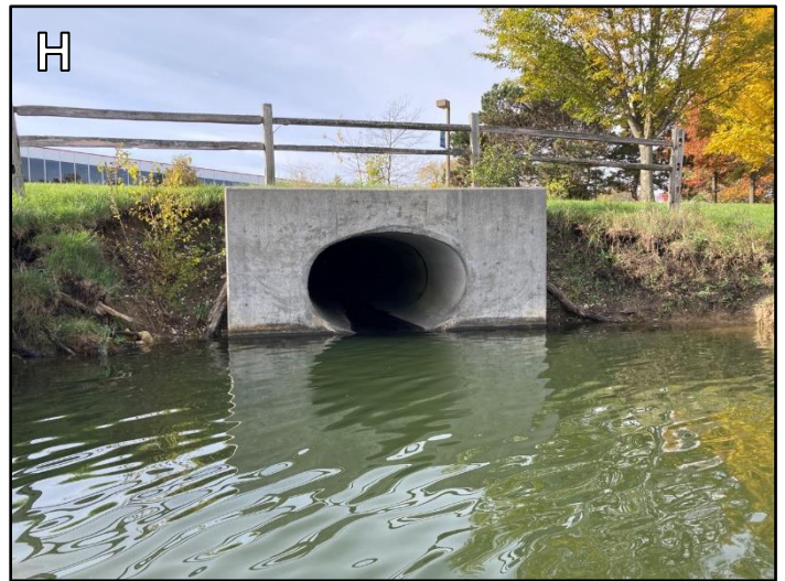
Photo 22. Erosion around culvert.
