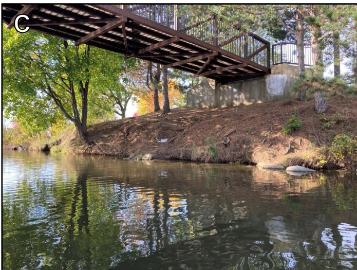
Photo 17. Severe erosion under bridge.
