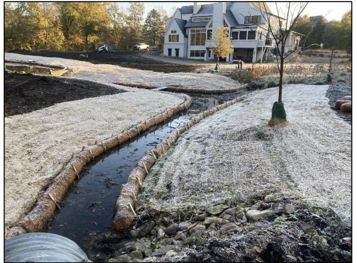
Photo 45. After – Stabilized with coir logs.
