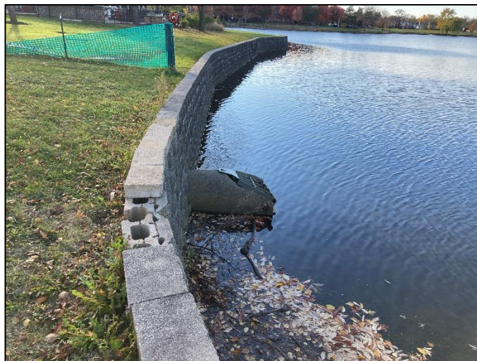
Photo 41. Missing seawall cap.
