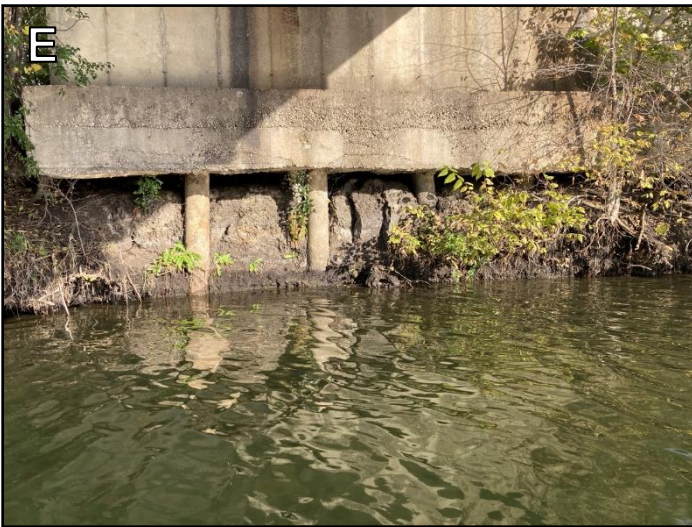
Photo 19. Severe erosion under bridge.
