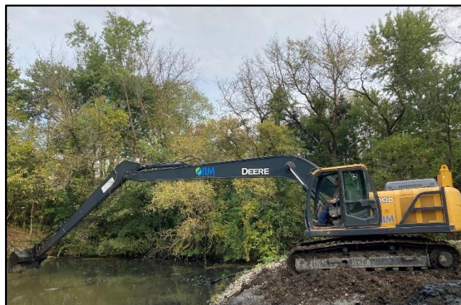
Photo 49. Mechanical dredging.
